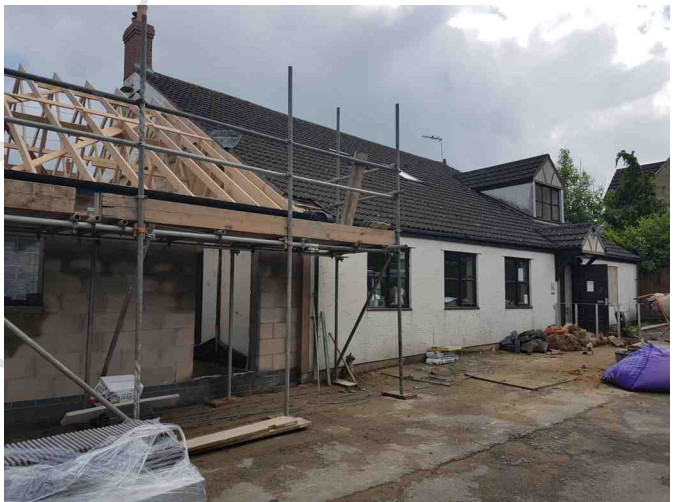
The new kitchen goes up
