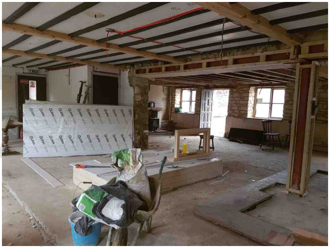
The wall between the two rooms is removed
